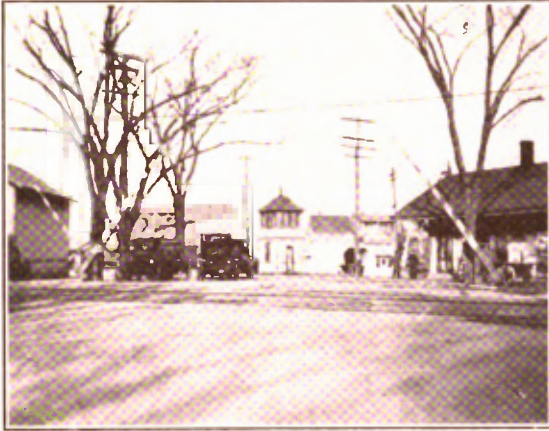
FIGURE 17.—Madison Avenue, one of the city's most important thoroughfares is cut in two at Ellison Street.
