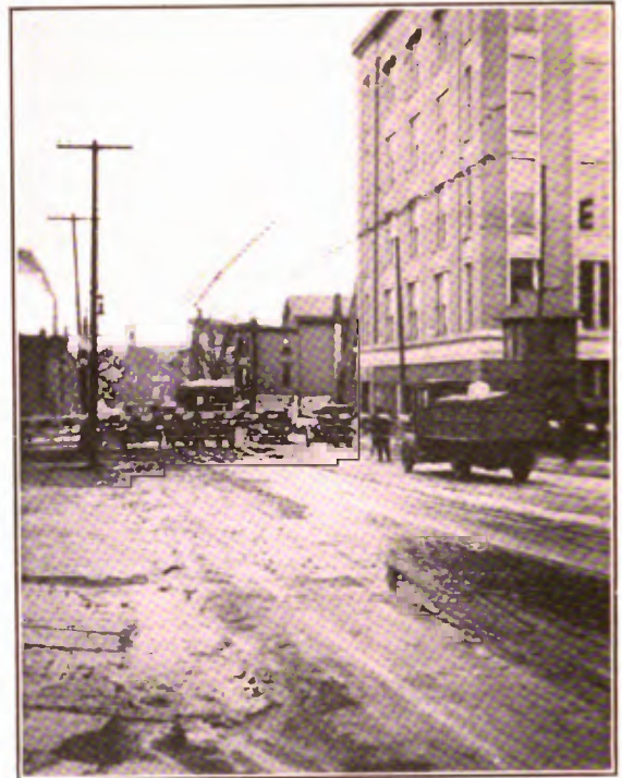
FIGURE 13.—While the railroad gates are down, all traffic waits.
