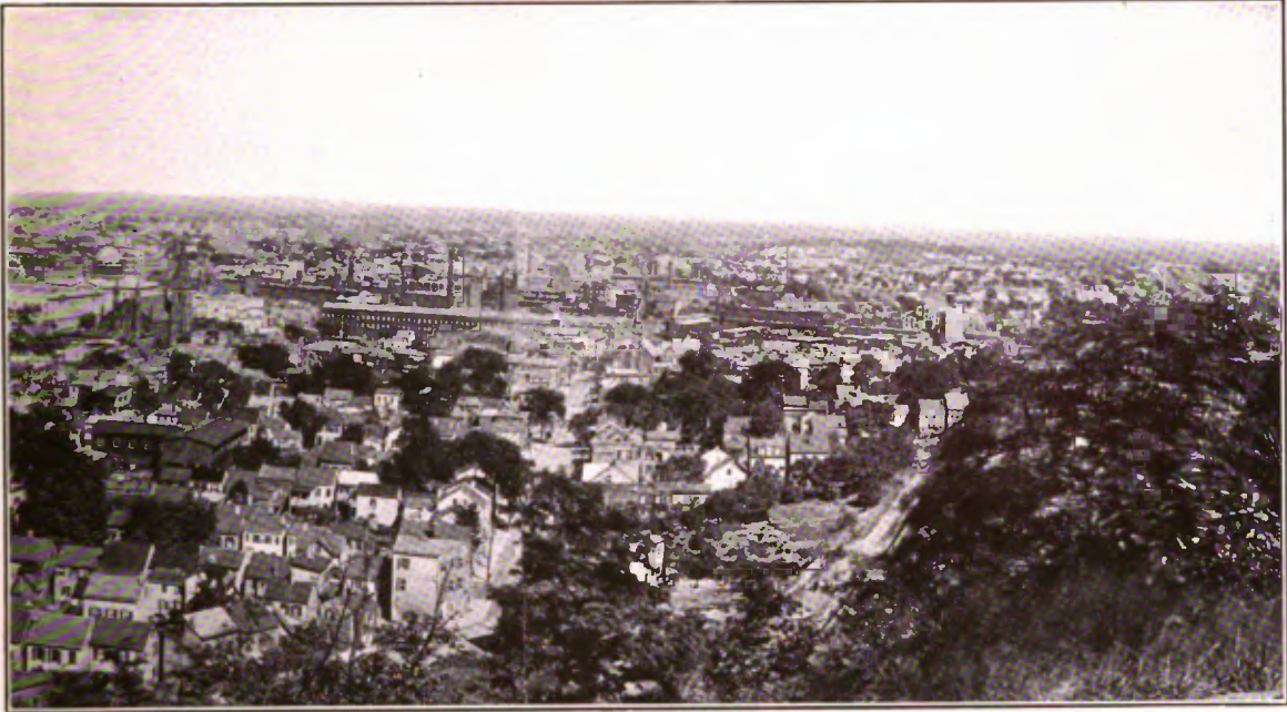
FIGURE 43. Downtown Paterson. Paterson is peculiarly blest among American cities in not having any high skyscrapers. The zoning law, moreover, limits the height of buildings to one and one-half times the width of the street with a maximum of 125 feet in the downtown section.
